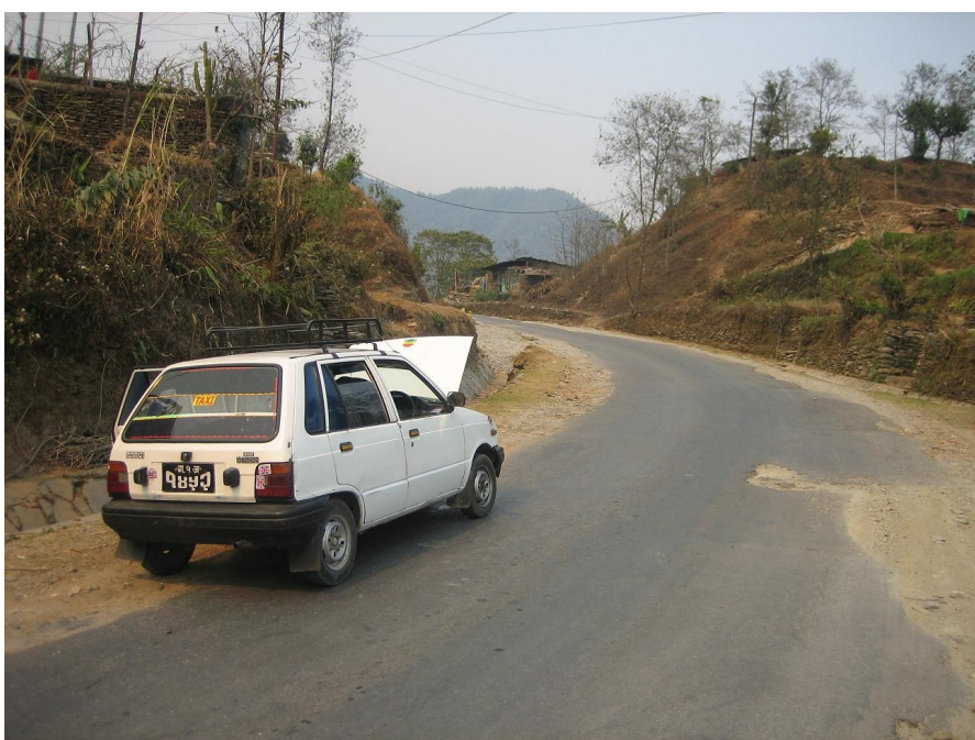
Figure 16 OUTSKIRTS POOR ROAD CONDITIONS; fringe of the KMC on the way to Pokhara (a sub metropolitan city) MARCH 2009 WALTER SUWAL
