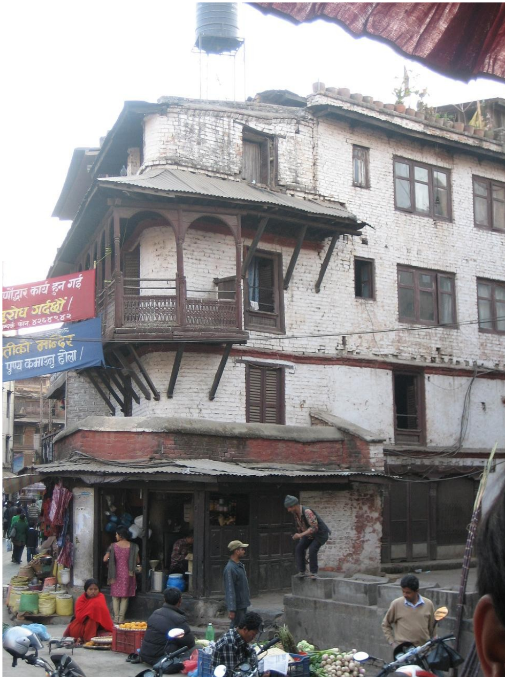
Figure 9 URBAN RESIDENTIAL AND COMMERCIAL; transitioning land uses MARCH 2009 WALTER SUWAL
